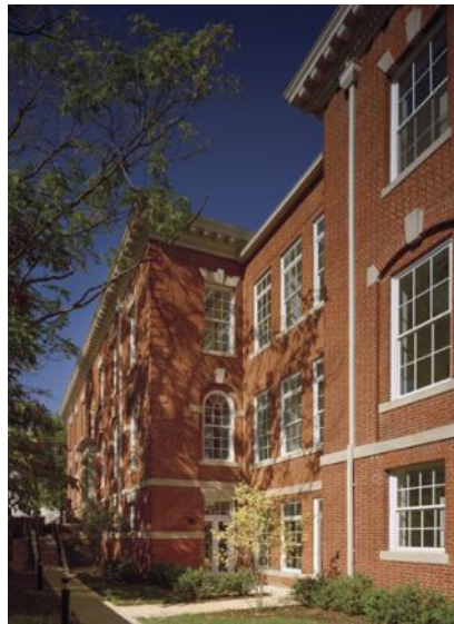
above: landmark in danger of demolition with partially collapsed roof; a hyphen infill accommodates a stair, elevator and additional bedroom space right: restored main entrance
