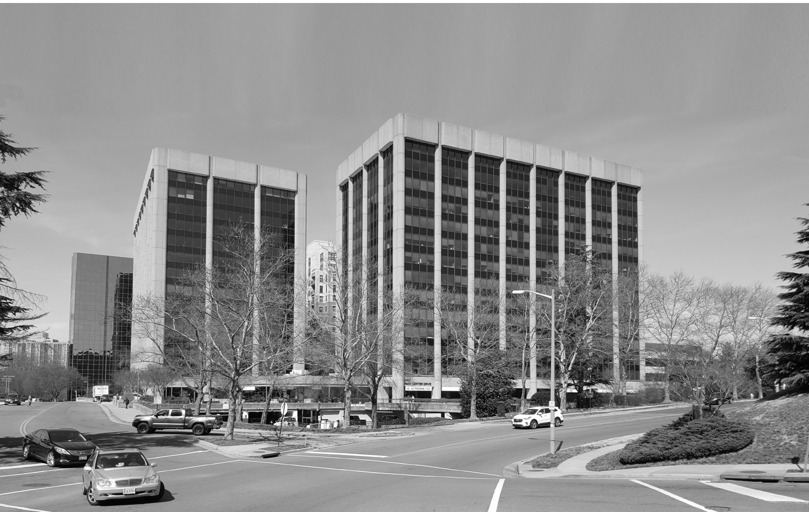
Before (above) and after (next page) of Park + Ford, a multifamily residential conversion of two existing 1980's office buildings in Alexandria, VA.
