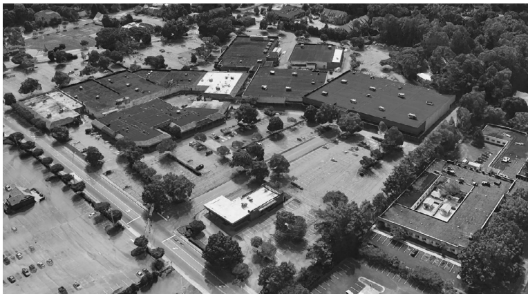
Before (bottom) and after site photos of Midtown Row
