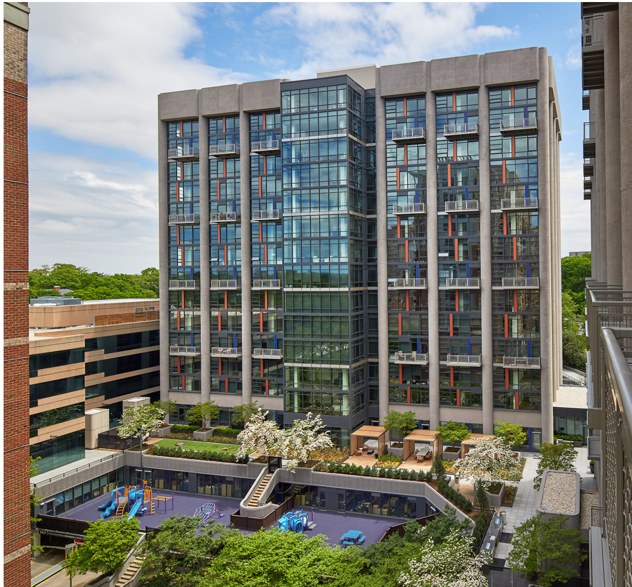
The original office bathroom core in Park + Ford became a glassy projected column bringing natural light into living spaces.
